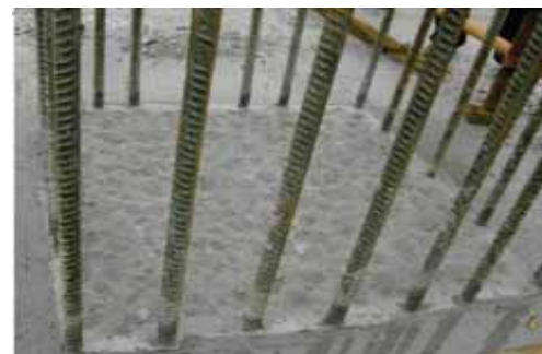
柱子施工缝
